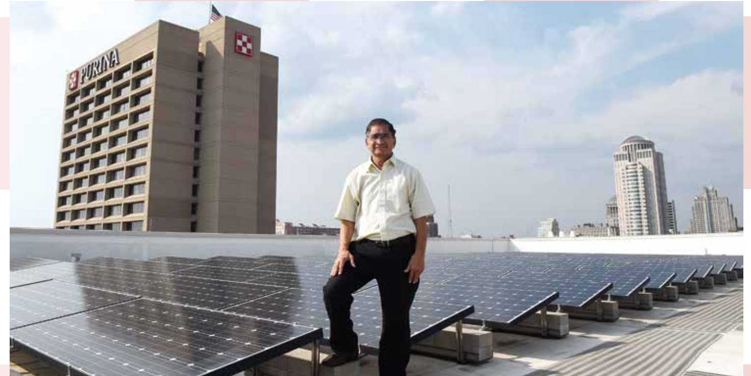
The roof of Nestlé Purina's newest Gold LEED building in downtown St. Louis houses rows of solar panels which help partially provide energy for lighting and water heating for the building.
