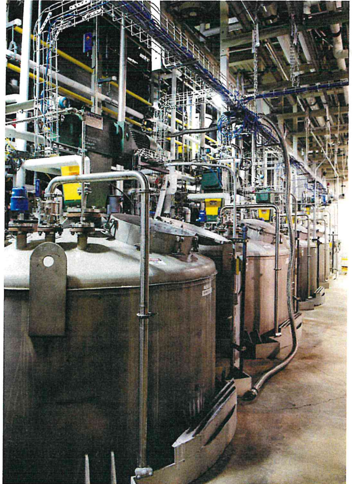
NCERC's Fermentation Alley includes four 22,000 liter bioreactors.
